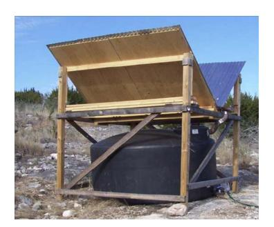
Final Assembly of Inverted Rain Collector
