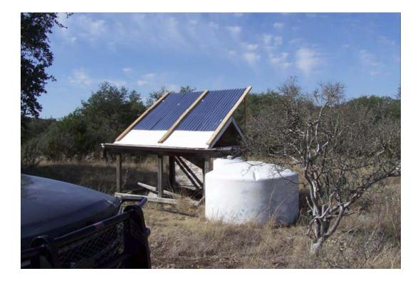
We have not had to truck water since we put in the new roof extension, but have not yet gone through a full summer with the new catcher either. We have now designed a single sided rain catcher that is efficient to build and that can be effectively used with a 550 gallon tank.
